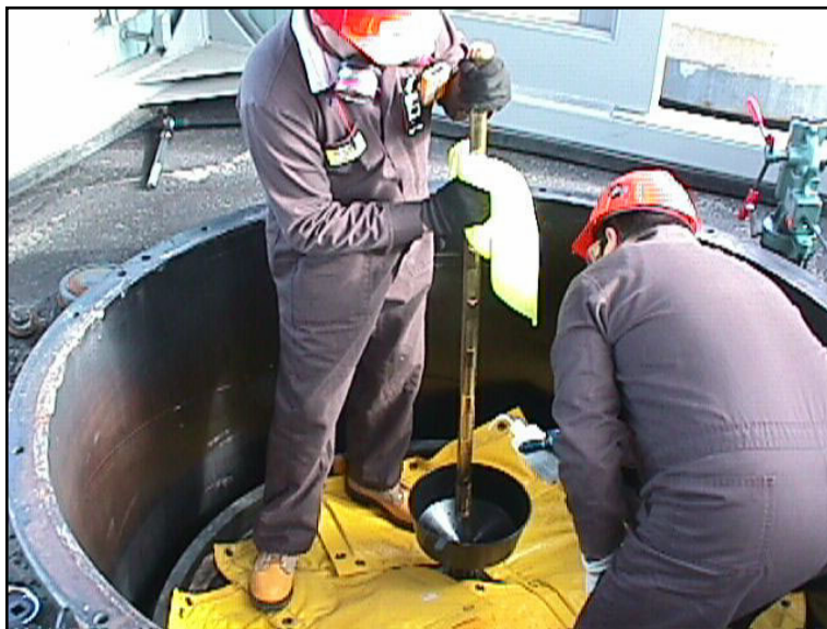
Figure 2. Resin Sampling from a Liner Stored Within an In-Ground Container
