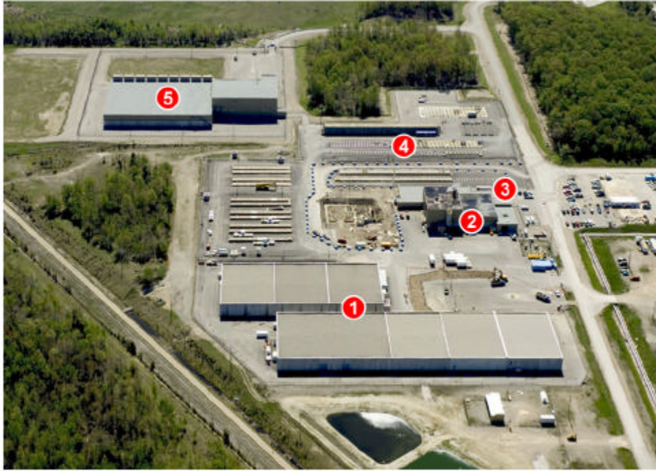
Figure 1: Aerial view of OPG's Western Waste Management Facility (May 2004); 1) Eight Low Level Storage Buildings with ninth under construction, 2) Waste Volume Reduction Building, 3) Amenities Building, 4) In-ground Containers, and 5) Western Used Fuel Dry Storage
