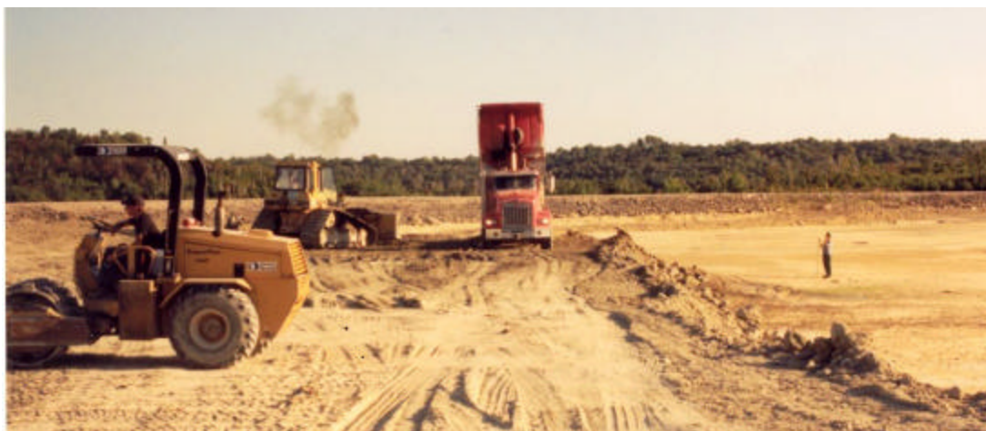
Photo shows till cover being applied at Cell 14
