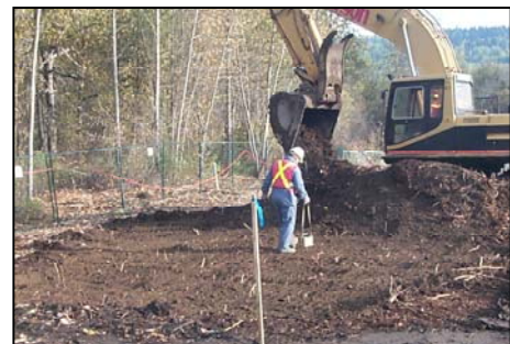
Contaminated Soil Identification and Excavation
