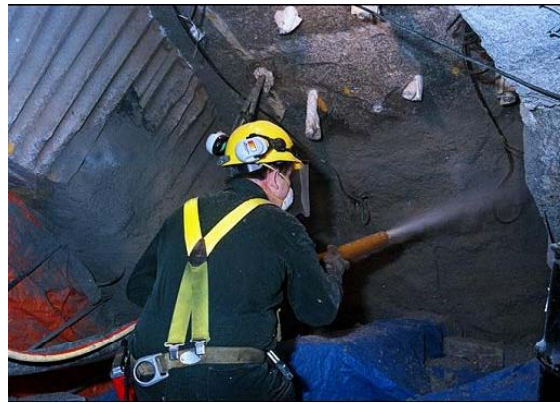
Figure 11: Application of Shotclay in the TSX and Backfill Wall
