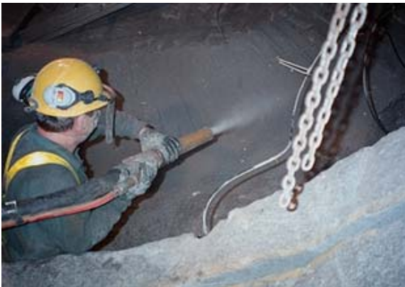
Figure 11: Application of Shotclay in the TSX and Backfill Wall
