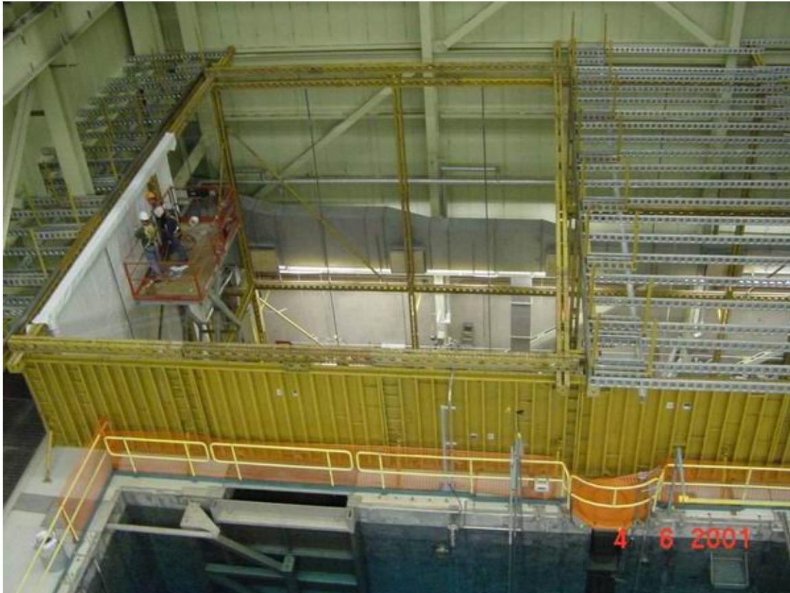
Fig. 4 The temporary environmental enclosure for concrete cutting/pouring.
