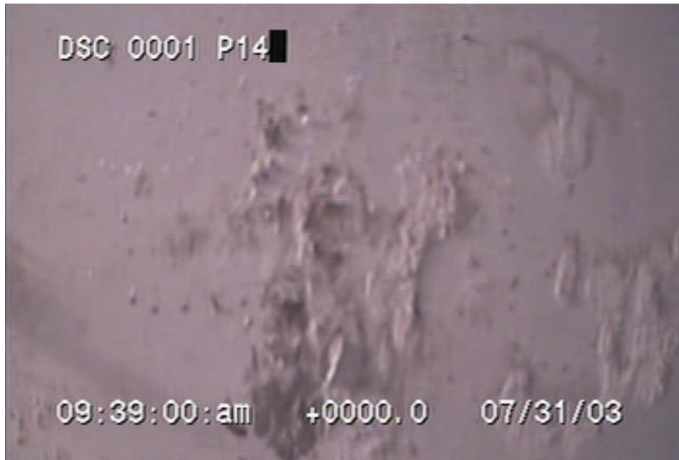
Figure 4 Damage to Coating Topcoat (typ.) (Scale: width = ~ 100 mm)
