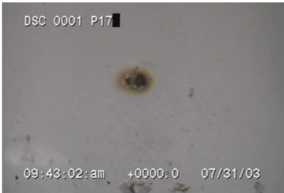
Figure 5 Surface Corrosion Where Coating Damaged to Steel (typ.) (Scale: width = ~ 100 mm)
