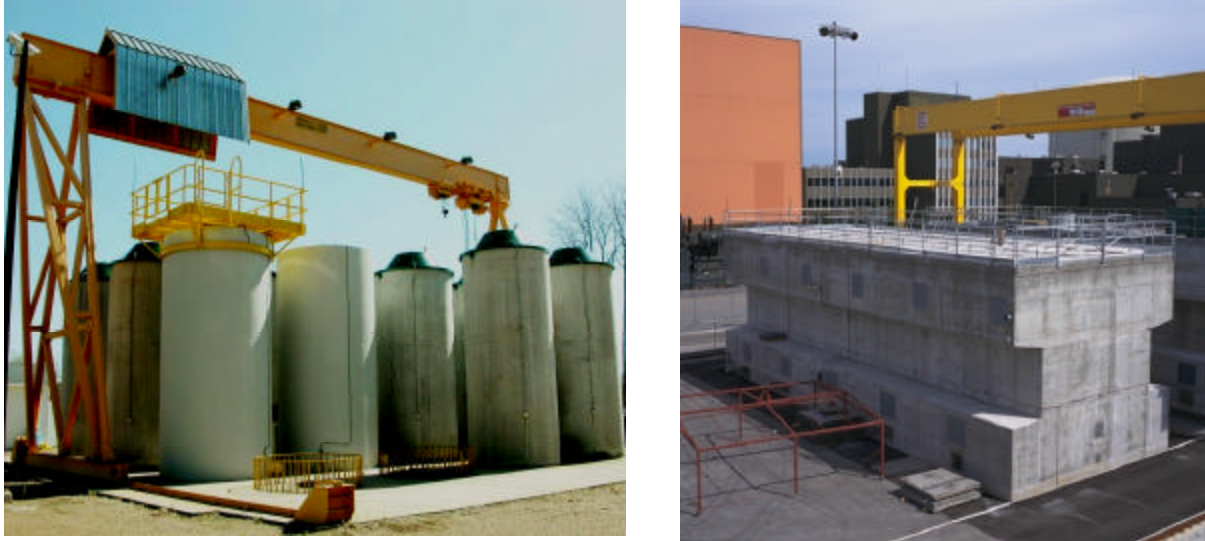
Figure 6. Concrete Canister Storage (left) for spent CANDU fuels at CRL, and Modular Air Cooled Storage (MACSTOR ® ) module at the Gentilly-2 reactor site (right).
