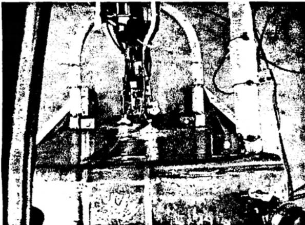
**Figure 14 :** Welding the final layer on the upper part of the mock-up.
