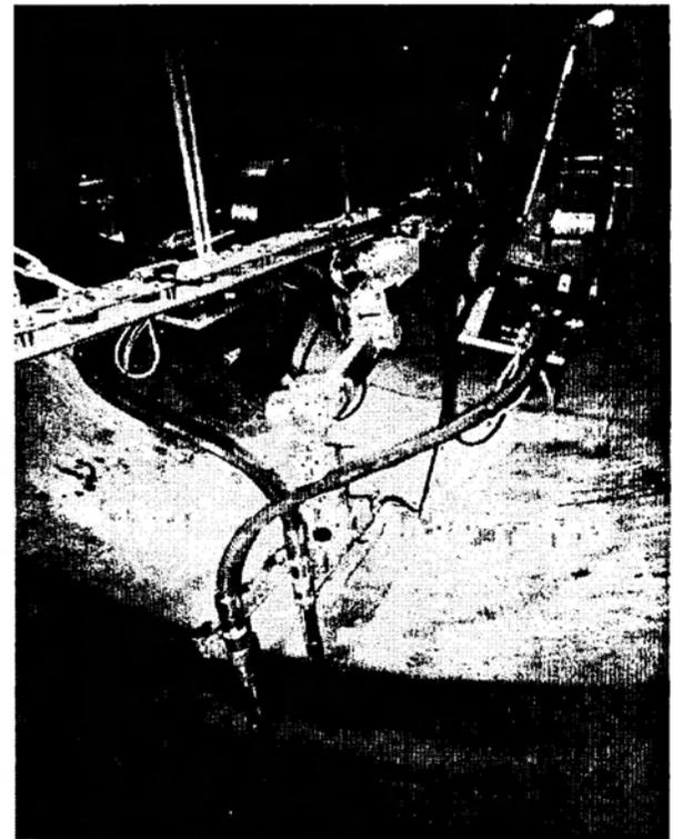
**Figure 7** : Tandem MIG overlay welding of the internal wall of an eroded carbon steel vessel :
