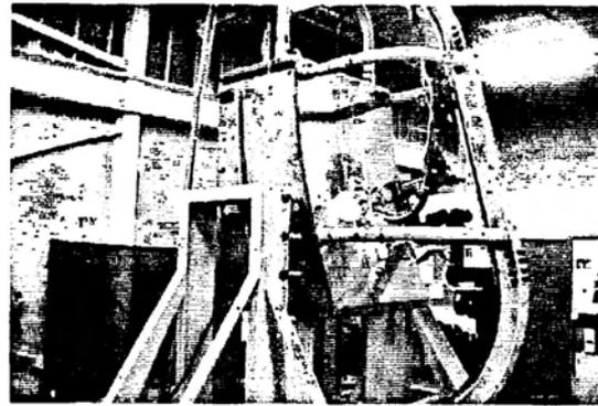
**Figure 15 :** Welding the final layer in the vertical position. The two robots are welding in tandem.
