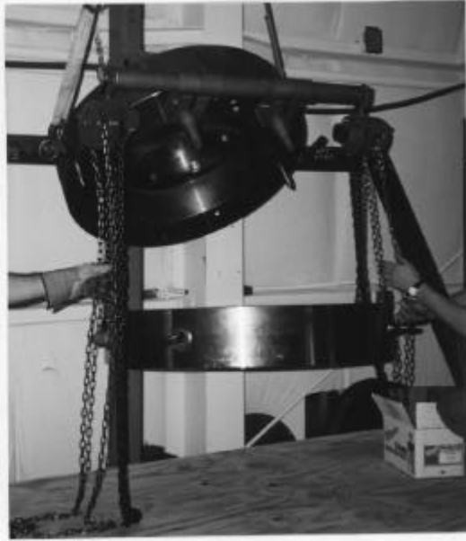
Figure 6 Chain Hoists Operated Simultaneously to Lower and Raise the Manway Cover
